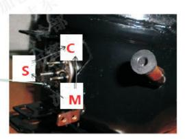
Normal range of C&M : About 10-30  $\Omega$ Normal range of C&S : About 10-32  $\Omega$ Normal range of S&M : About 20-60  $\Omega$ If the measure result is not in the range,it means the compressor has problem, change the compressor.
